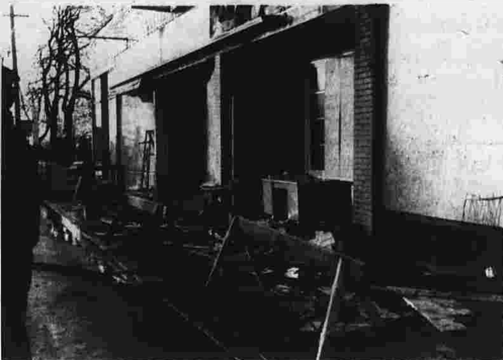
Firemen worked Sunday to help tenants of the Prichard block on Union Street, Rockville, salvage a few of their belongings in the aftermath of a fire that extensively damaged six of the eight businesses in the block. (Herald photo by Richmond)
